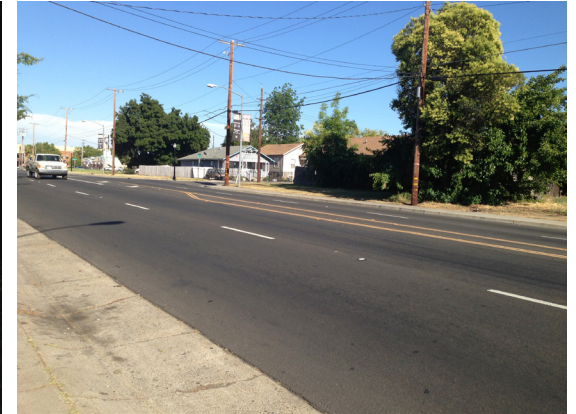
Figure 6.19 Travel lane and no bike lane
