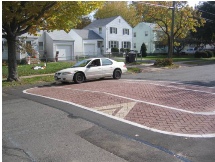
Figure 6.24 Speed table
