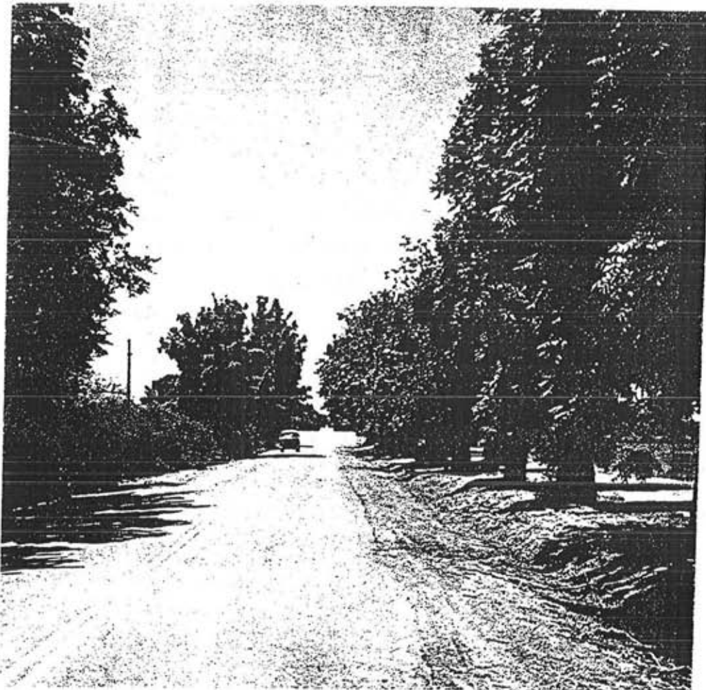
Connector Greenway (Road 98, looking north)
