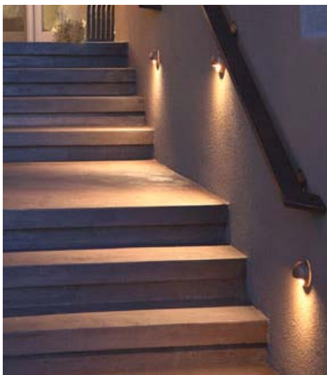
Example of stair lighting
