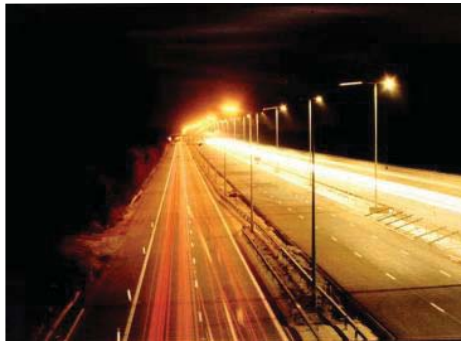
High Pressure Sodium lamps
