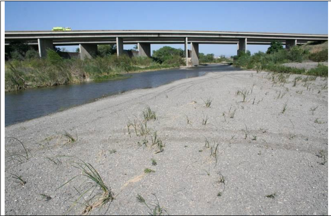
Figure 15 Highway I-505 Bridge from downstream
