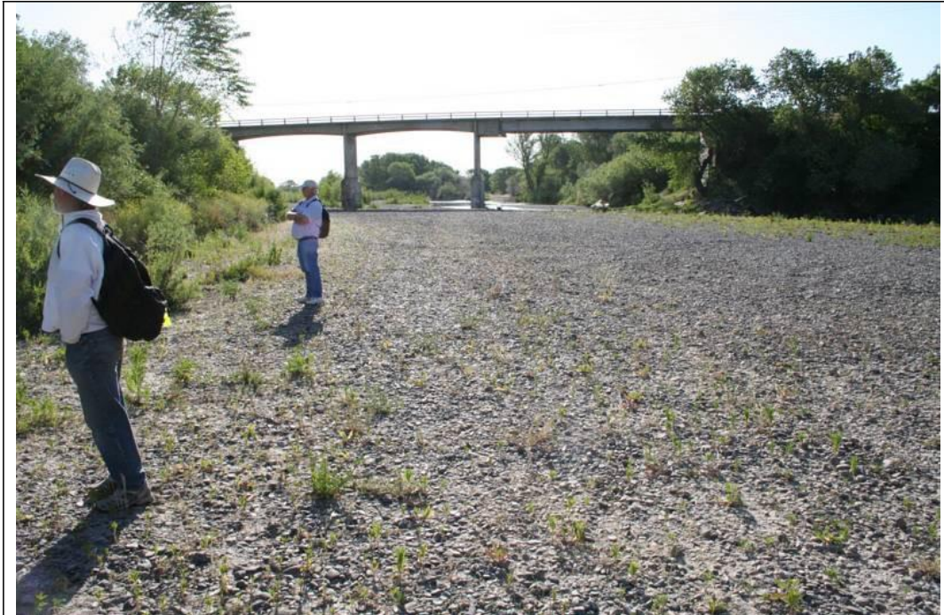
Figure 17 Bridge at Road 94B looking downstream
