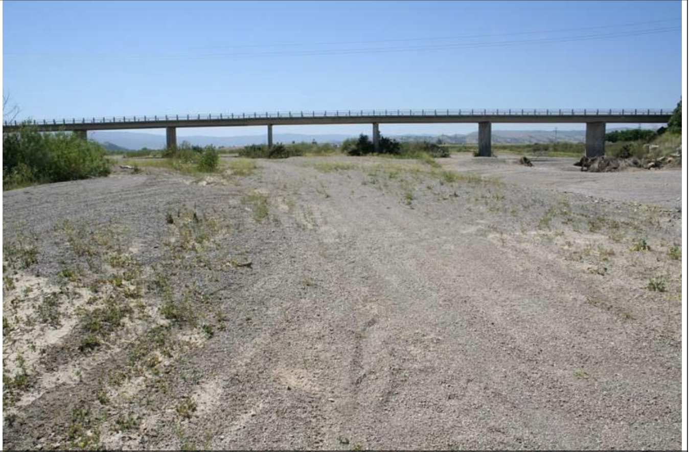
Figure 12 Esparto Road 87 Bridge
