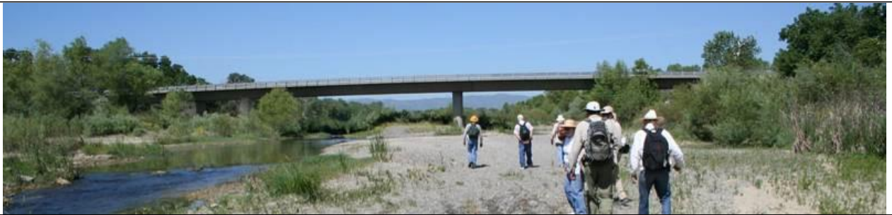
Figure 10 Capay Bridge - view from downstream
