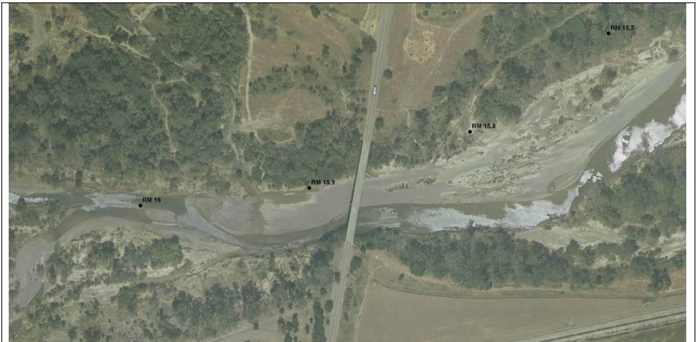
Figure 18 Bridge at Road 94B showing little constriction
