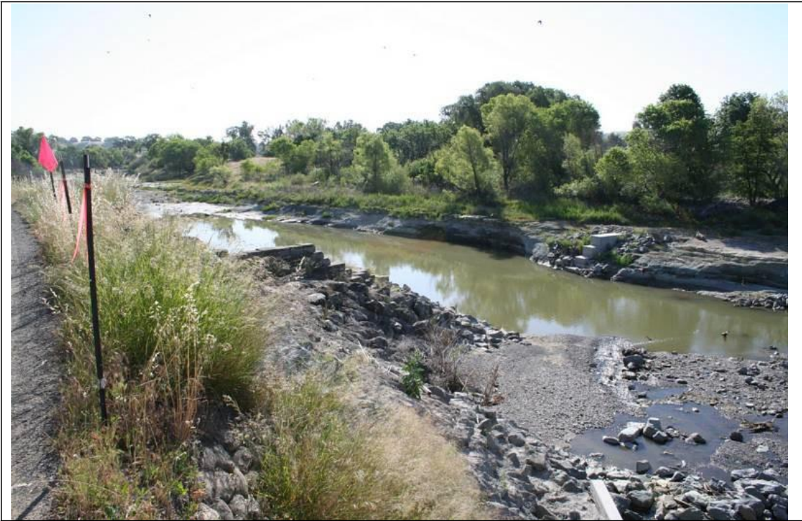
Figure 1 Grade control structure downstream of Capay Dam
