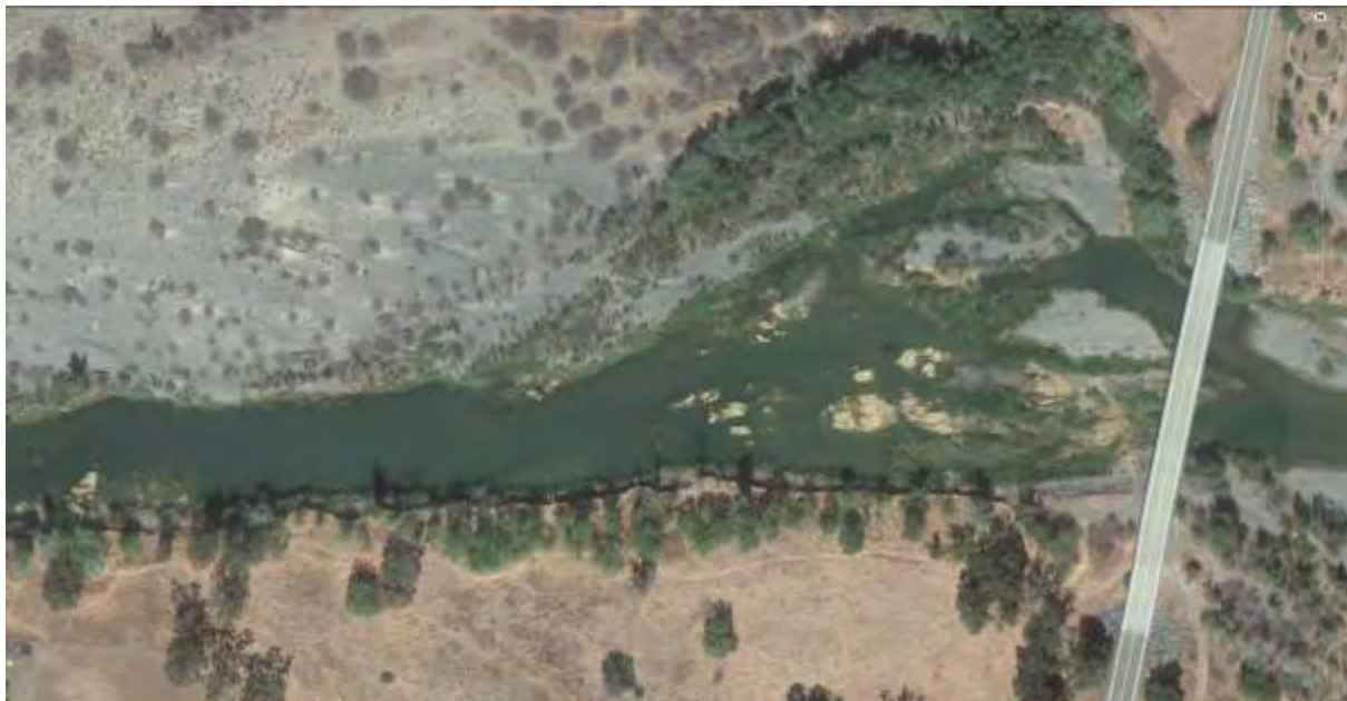
Figure 55 Capay Bridge (County Road 85) River Mile 26.35
