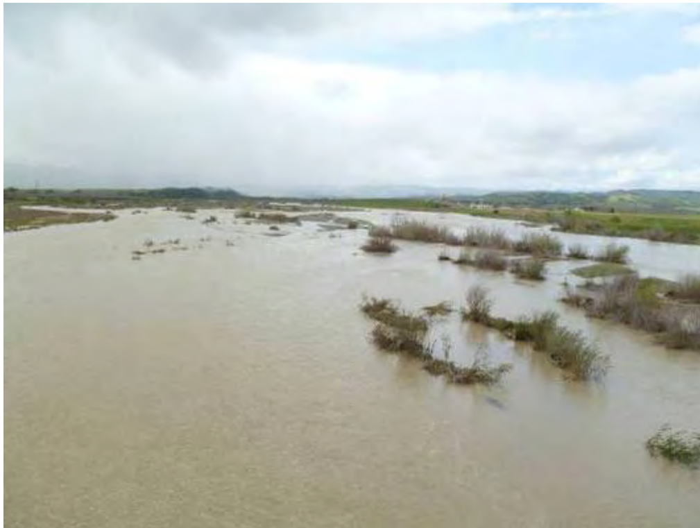
Figure 8 b From Esparto Bridge looking upstream
