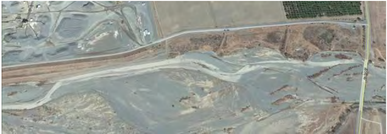
Figure 59 a Esparto Bridge (County Road 87) River Mile 24.4
