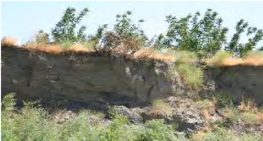
Figure 34 Active erosion at RM 21.6 north bank (2008).
