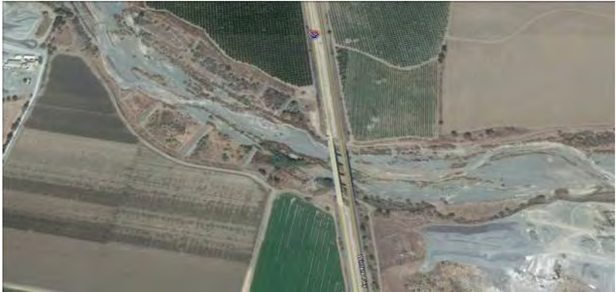
Figure 64 Interstate 505 Bridge (River Mile 21.0)
