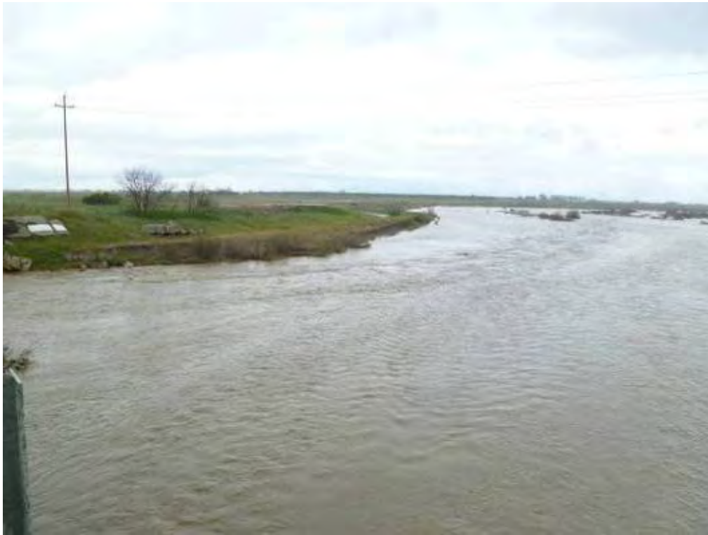
Figure 8 c From Esparto Bridge looking downstream
