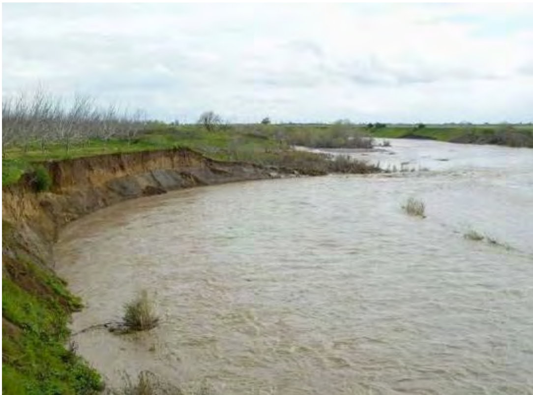
Figure 39 Road 84b Bridge site looking downstream (2011)
