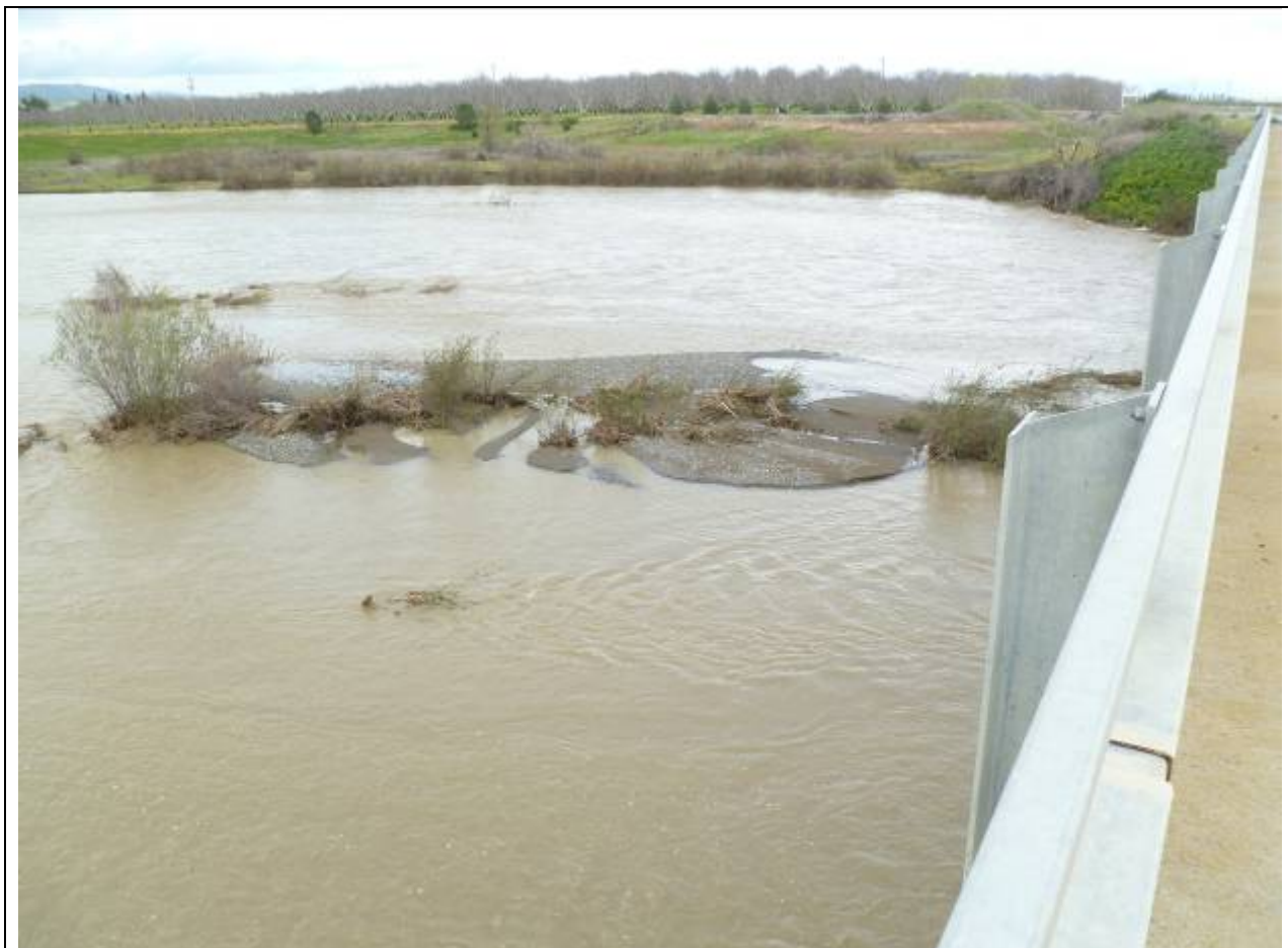
Figure 1 Photo of new channel deposits from Esparto Bridge County Rd 87 at flows of 5,000 to 6,000 cfs
