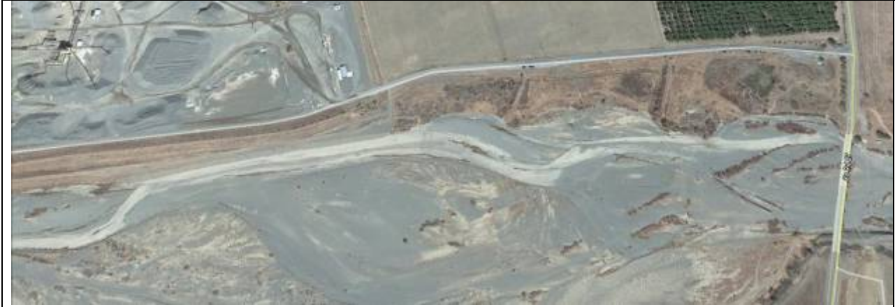
Figure 32 Esparto Bridge (County Road 87) River Mile 24.4
