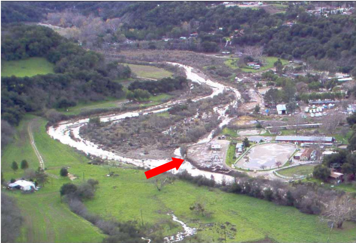
Figure 1. Oblique Photograph of the Project Area Looking Downstream with an Arrow Indicating the Fill that Diverted Flow to the Left Bank Just Prior to the January 2005 Storm.
