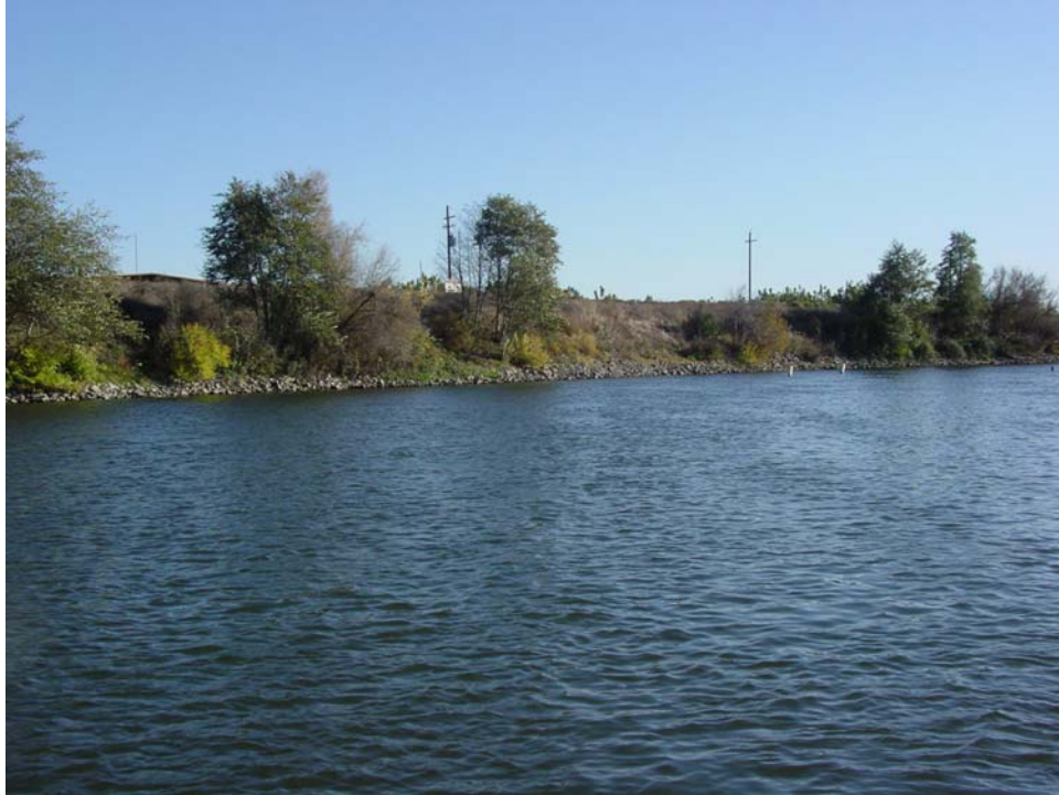
Plate I-4 View of eroding bank at RM 193.5R.
