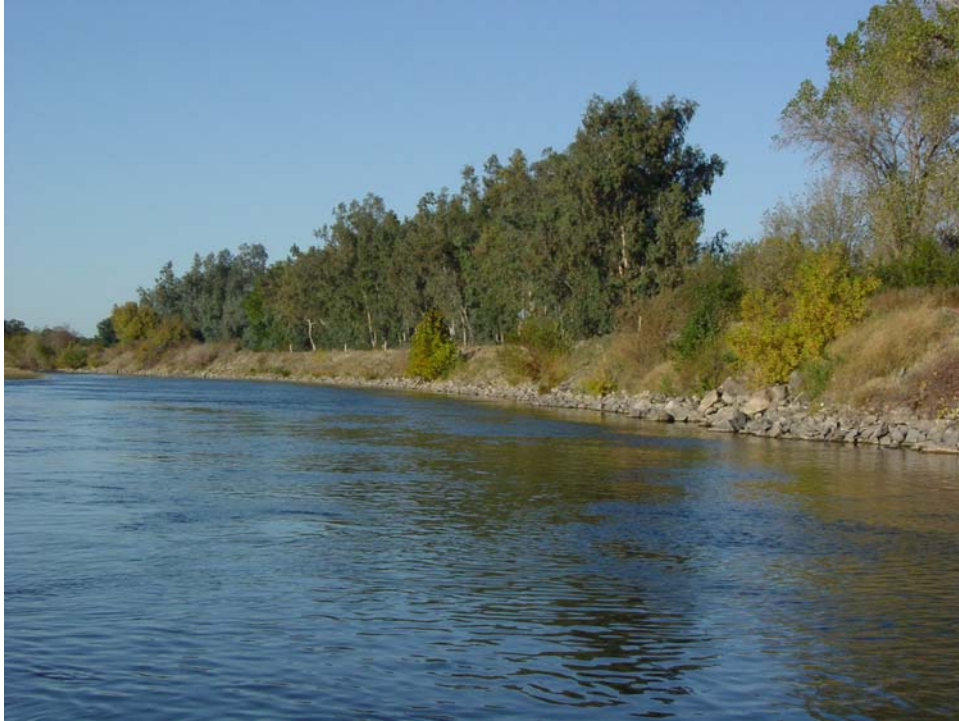
Plate I-2 View upstream of revetment at about RM 194L.
