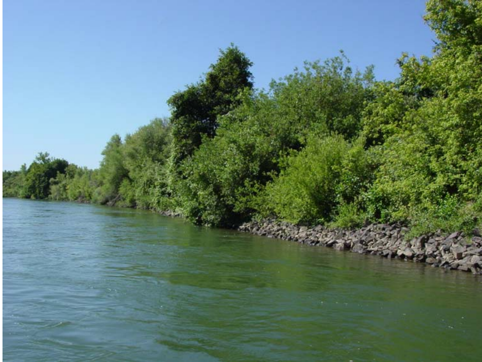
Plate I-1 The Sacramento River, view downstream of revetment at about RM 198R.
