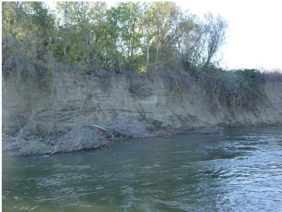
Plate I-3 View downstream of revetment at RM 193L.
